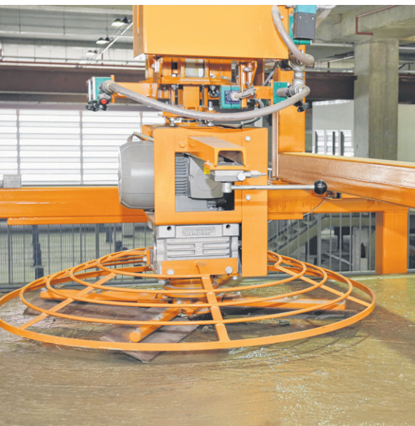
5 A machine smooths the precast surface.
