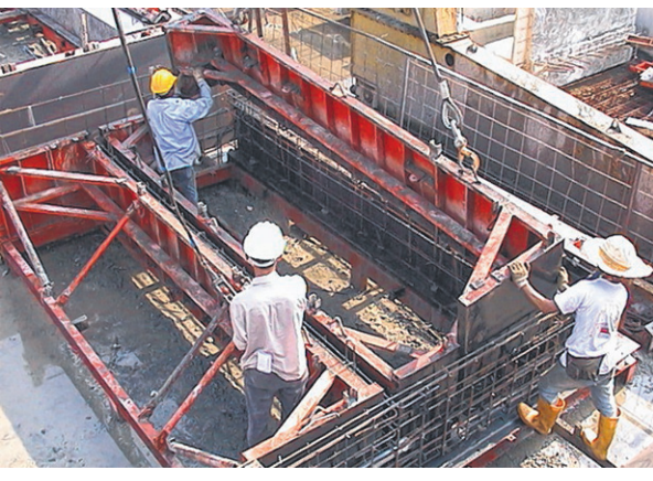
1 Workers assemble the mould in the required shape.
