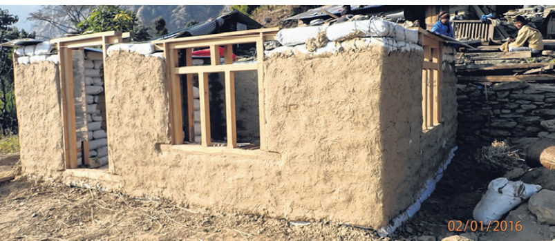
3. The wall is plastered with materials like mud or clay.
