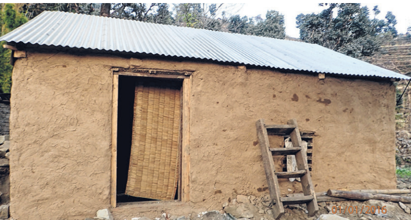
4. A roof made of zinc or straw is placed on top.
