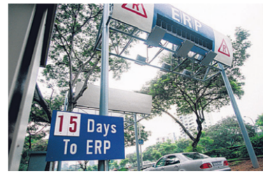
Rolled out on April 1, 1998, the ERP system automated toll payment and collection.
