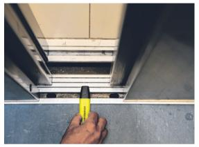
• Checking the lift car doors This includes testing that the lift will not move if the doors are more than 25mm apart.
