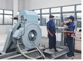
Checking the traction machine, which is what makes the lift run, in the motor room
