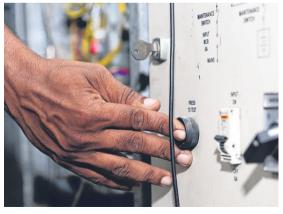
• Testing the emergency battery-operated power supply
