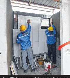
The PBUs are completed with finishes such as copper piping (inset), partial tiling, window frames and a waterproofing system.
