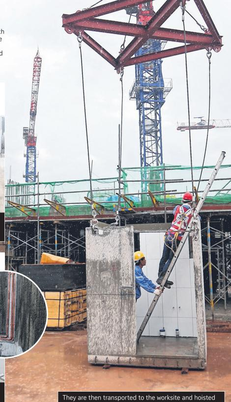
onto the blocks for installation.
