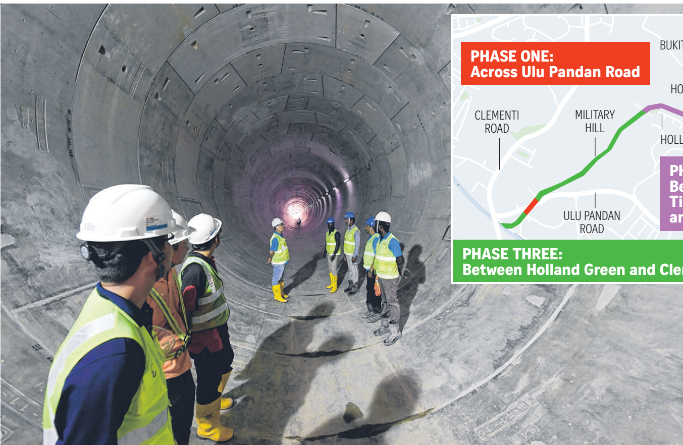
(Left) One of the two new tunnels being added to a segment of the Bukit Timah First Diversion Canal, which runs from Holland Green to Clementi Road. The tunnel will help to take in rainwater from the Upper Bukit Timah catchment, and help to prevent flooding in the area.
