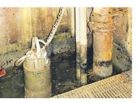
The lowest float switch, which would have activated the storm water sump pumps, was impeded by accumulated silt and sludge in the Bishan storm water sump pit.
