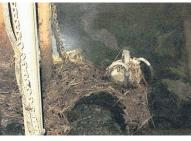
Floating debris in the pit could have impeded the normal functioning of the float switches, in particular the highest float switch, which alerts SMRT's Operations Control Centre to high water
