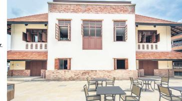
Terracotta and fairfaced brickwork set against rough textured plaster were reinstated and the original foyer spaces were retained. • The original French windows, timber shutters and lattice vents were reintroduced to the structure as well.
