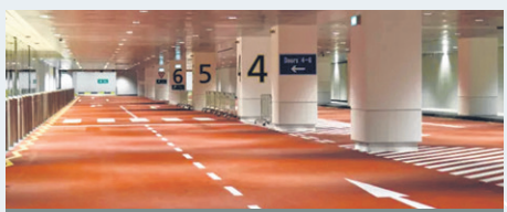
There will be separate driveways for Jewel and T1 where a new driveway (above) recently opened.
