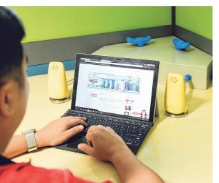
This personalised ventilation system delivers fresh air directly to each occupant through pipes attached to a desk. which resemble speakers. This reduces energy usage because there is no longer a need for the entire floor or room to be cooled to a low temperature.
