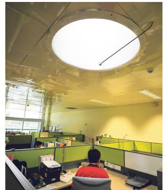
Light pipes set up on the building's roof collect sunlight and, through reflection via mirrors, throw this harvested daylight into the room below. The light is spread evenly throughout the room by diffusers. reducing the need for artificial lighting.
