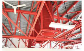
Specially developed for tropical climate, solar chimneys are made of metal that absorbs solar radiation. Placed on top of the roof or up high in a nonair-conditioned room, they suck out warm air from the room. Through convection, cool air will then rush into the room.
