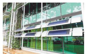
Strategically placed shading contraptions can shield the building from the sur while bouncing natural lighting into the interiors of the building. And plants planted vertically on the walls can shade them from the sun and lower indoor temperatures.
