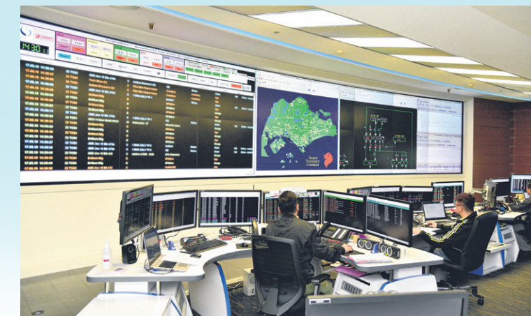
SP Group's distribution control centre where monitoring of the power grid and remote switching is done.
