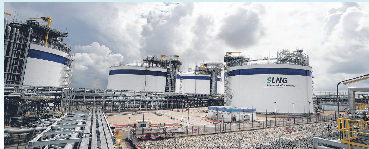
The Singapore LNG Terminal located on Jurong Island is Singapore's only liquefied natural gas terminal.
