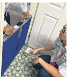
A lever is used to extend the side panels 2 until it touches the door frame
