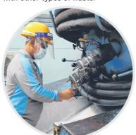
Greasy waste is piped from the tankers into a pre-treatment facility.
