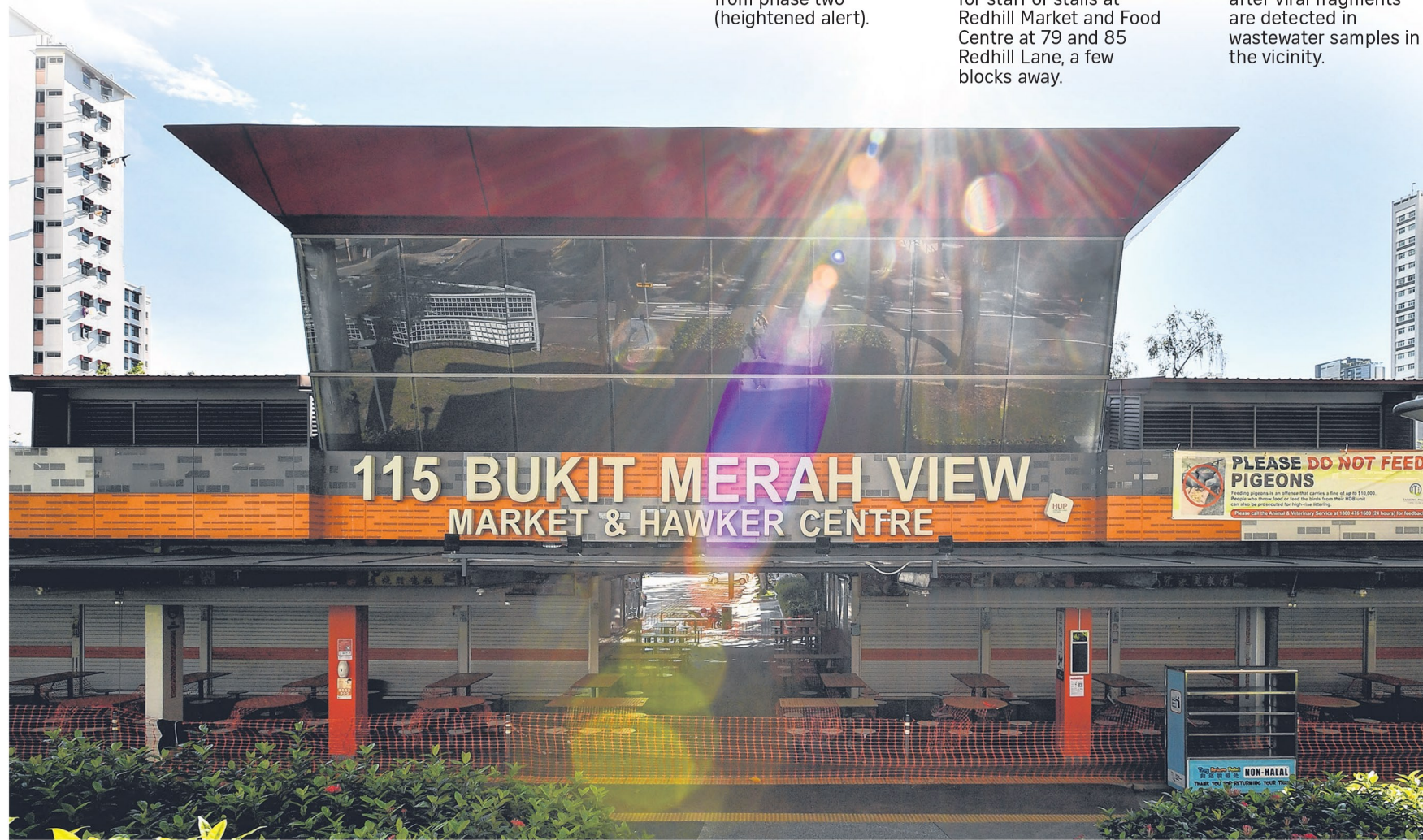
The site of Singapore's largest open infection cluster remains closed till Saturday.
