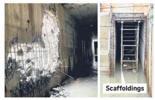
3 But the diversion drain was not properly connected to the existing drain and was partially obstructed by scaffoldings.
